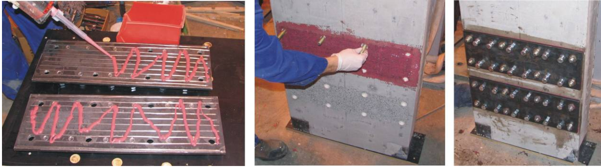
Figure 9. Damper connection details; Left: Preparation of the steel plate – roughening and application of high strength epoxy, Centre: Roughening of the concrete, application of high strength epoxy and location of the high strength threaded rods, Right: Installation of the steel plates - threaded rods tightened to 65% proof load.
