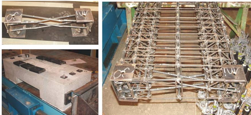
Figure 7. Construction of the precast wall unit and precast foundation; Top Left: Steel confining plates, Bottom Left: Precast foundation, Right: Wall reinforcement.
