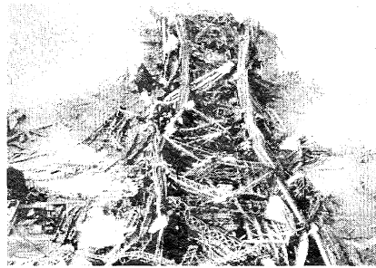
Cooper's Quebec Bridge after collapse
