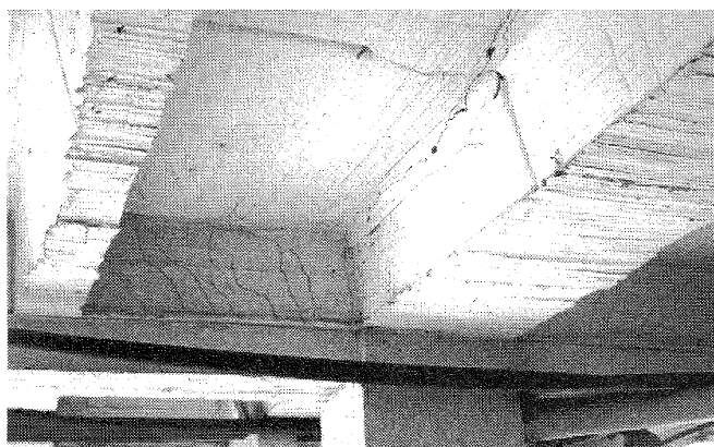
Figure 28: Positive and negative plastic hinges in a gravity dominated beam of a reinforced concrete frame (Veraneros Courts).
