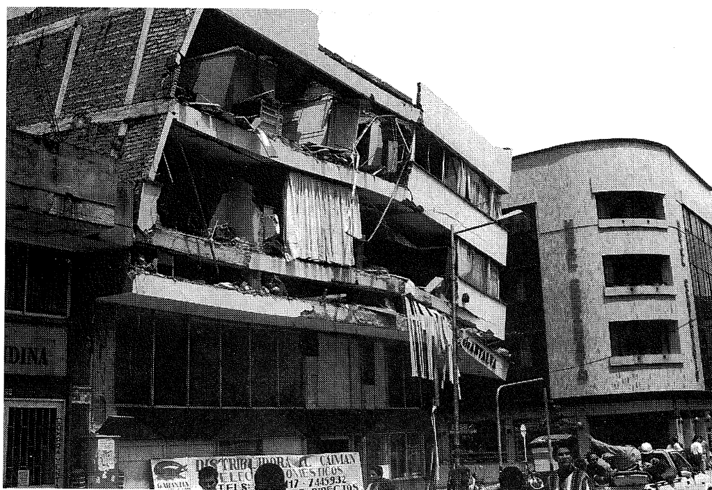
(a). Intermediate soft storey mechanism in Artalva Courts, Armenia, caused by the collapse of the infill walls. (Courtesy of E Castrillon).
