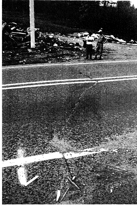
Figure 4: Right-lateral displacements at a road margin near the town of Barcelona.
