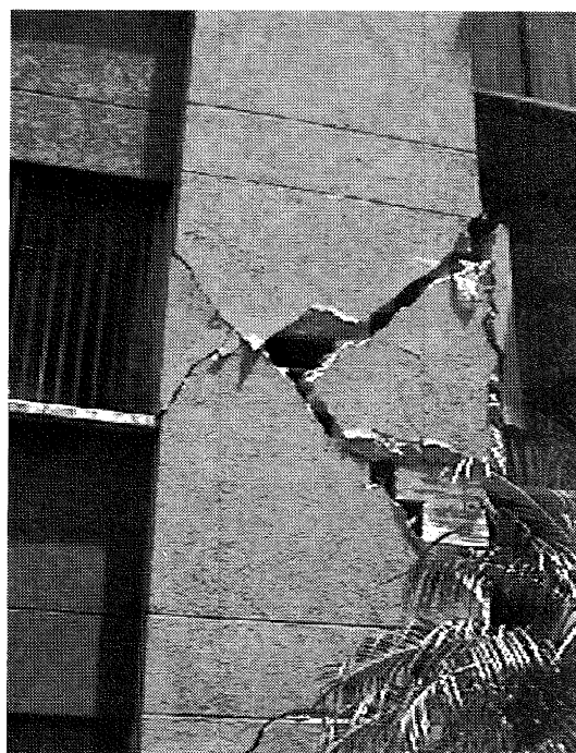
(c). Non-structural damage to a clay brick façade.
