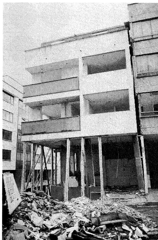
Figure 24: Excessively displaced corner building in Pereira.
