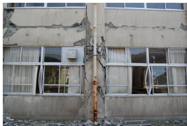
Figure 2: Damage due to non-structural walls during the 2011 Tohoku Earthquake.
