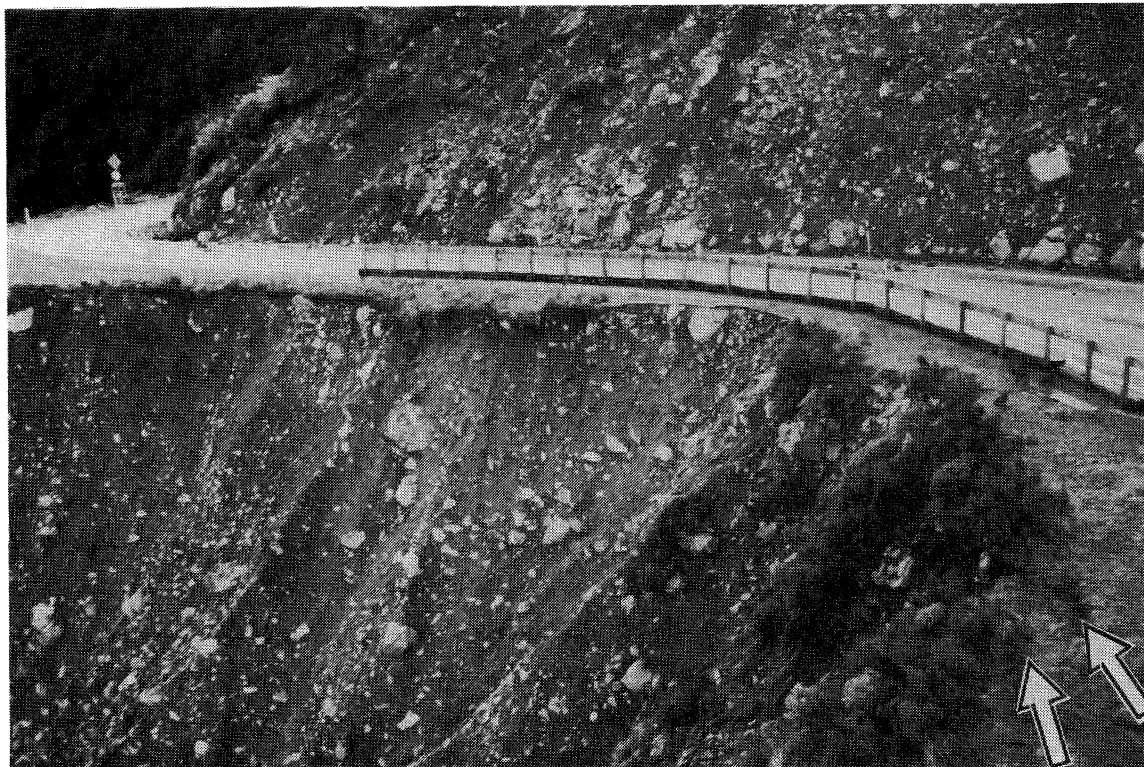
FIGURE 9 Tension cracks (bottom right) along the edge of oversteepened slope at the top of the Zig Zag.
