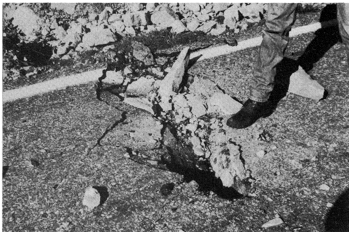
FIGURE 4 Impact crater on the highway near the top of the Zig Zag.
