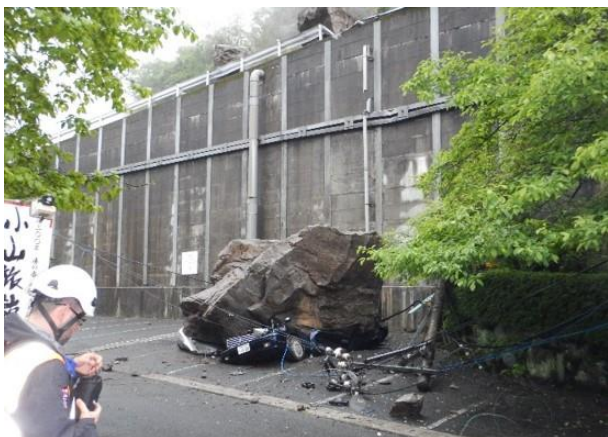
Photo 31: Good performance of a tied-back retaining wall with EPS backfill (N 32.8711; E 130.9916).
