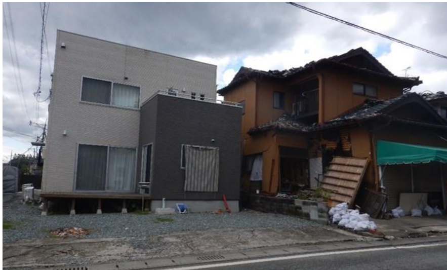
Photo 2: Low damage to a new residential house (without tiled roof) and severe damage to two-storey timber house (with heavy tiled roof) observed in Mashiki Town (N 32.7876; E 130.8185).
