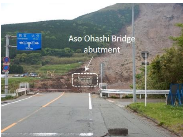
Photo 42: Landslides caused the collapse of a number of bridges in the mountainous areas of Mt. Aso volcanic caldera (N 32.8834; E 130.9896).
