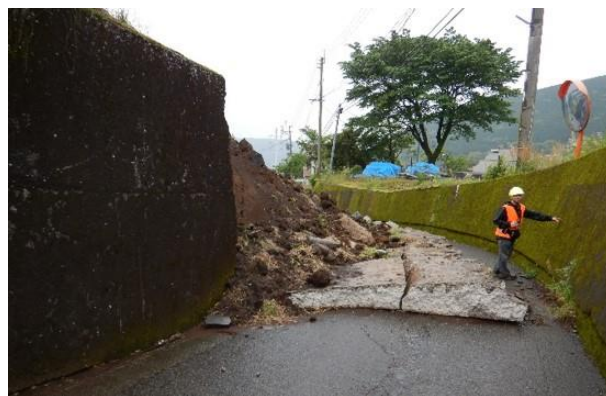
Photo 27: Complete collapse of a typical unreinforced concrete wall in Minami Aso Village (N 32.8844; E 130.9918).
