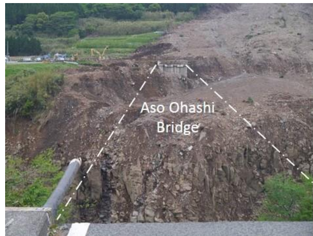
Photo 16: Toe of the debris avalanche at Aso Ohashi Bridge. Note the bridge has been destroyed by the landslide (Location 10 in Figure 2: N 32.8834; E 130.9896).
