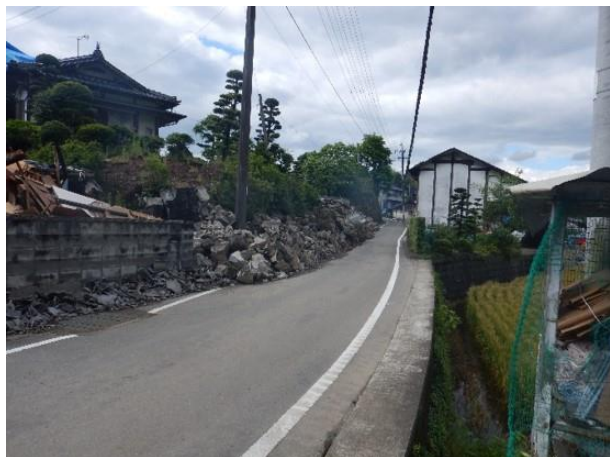
Photo 25: Collapse of a typical unreinforced wall in Nishihara Village (N 32.8056; E 130.8583).
