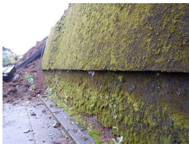
Photo 28: Displacement of the upper part of a wall along construction joint (N 32.8843; E 130.9916).
