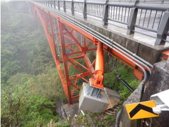
Photo 46: Connection of a retrofitted damper of steel arch bridge failed at one abutment (N 32.8779; E 130.9094).
