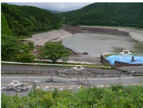
Photo 4: Surface fault rupture at the Ookirihata earth dam in Nishihara Village (Location 23 in Figure 2: N 32.8415; E 130.9321).
