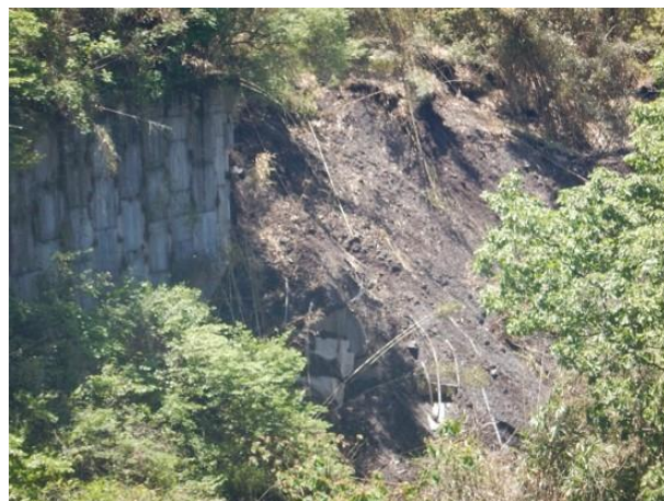
Photo 29: Total collapse of a reinforced earth wall near Tokyu Country Town (N 32.8805; E 131.0039).
