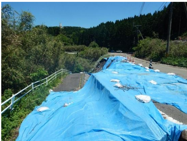
Photo 30: Effects of the collapse of the reinforced earth wall (shown in Figure 29) on the supported road (N 32.8804; E 131.0040).
