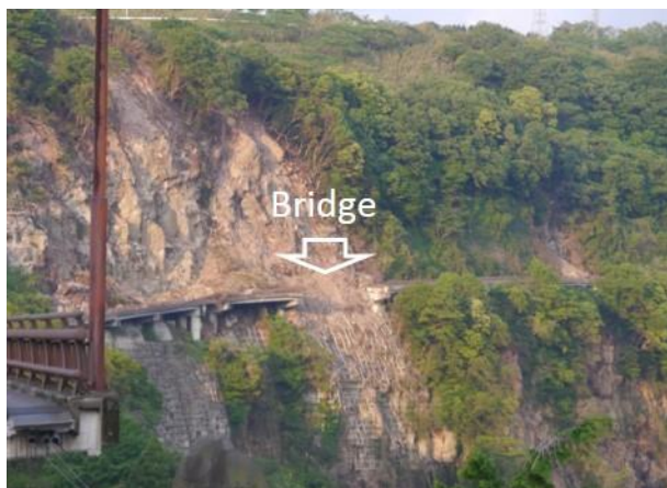
Photo 17: Bridge deck destroyed by a relatively small debris avalanche (N 32.8752; E 131.9886).
