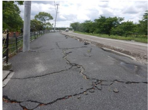
Photo 24: Cracking, lateral displacement and tilting of power lines induced by lateral spreading in Mashiki Town (N 32.7860; E 130.8177).
