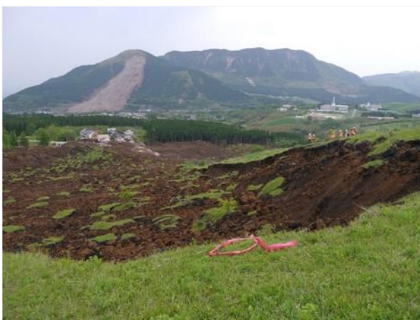
Photo 6: Source of earth flow/slide in Minami Aso Village (looking downhill), with damaged houses and the large debris avalanche at Aso Ohashi Bridge visible in the distance (Location 9 in Figure 2: N 32.8851; E 131.0049).
