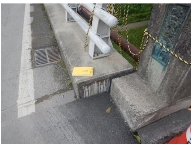
Photo 37: A two span bridge jumped 300 mm laterally off its bearings (view from the road) (N 32.7864; E 130.8186).
