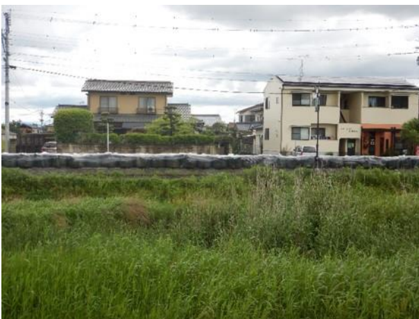
Photo 23: Temporary flood protection measure to mitigate the impact of liquefaction-induced subsidence of river bank in Mashiki Town (N 32.7832; E 130.8084).
