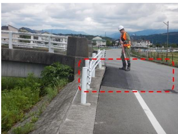
Photo 36: Temporary ramp being formed to provide access due to settlement of short span concrete bridge approaches (N 32.7830; E 130.8085).
