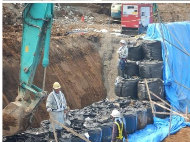
Photo 48: Collapse of a retaining wall supporting an expressway embankment. Gravel filled polyester bags were used to quickly rebuild the wall and reopen the expressway (N 32.7792; E 130.7943).
