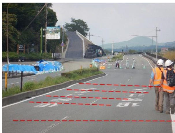
Photo 34: Some cracking appeared on the road supported by the walls shown in Photo 33 (N 32.8792; E 130.9833).
