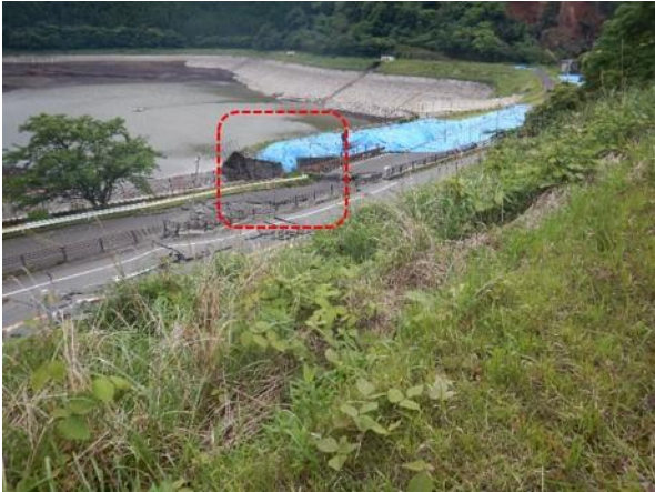
Photo 50: Fault rupture damaged the spillway of the Ookirihata earth dam (N 32.8414; E 130.9317). See also Photo 4.
