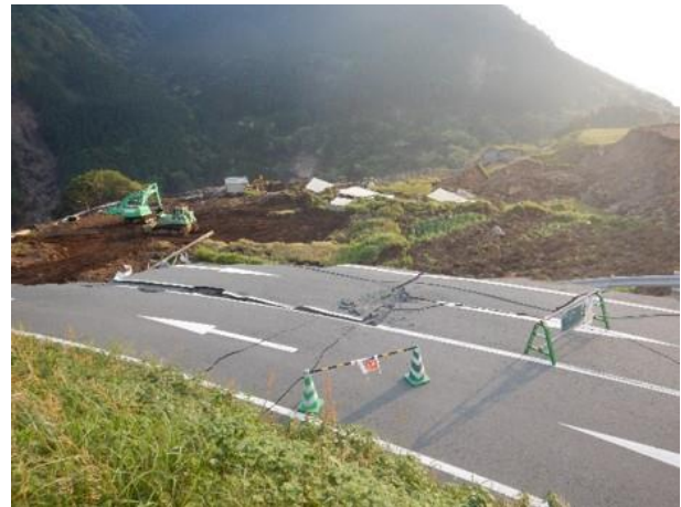
Photo 52: New dam construction site destroyed by fault rupture (N 32.8776; E 130.9764). See also Figure 20.
