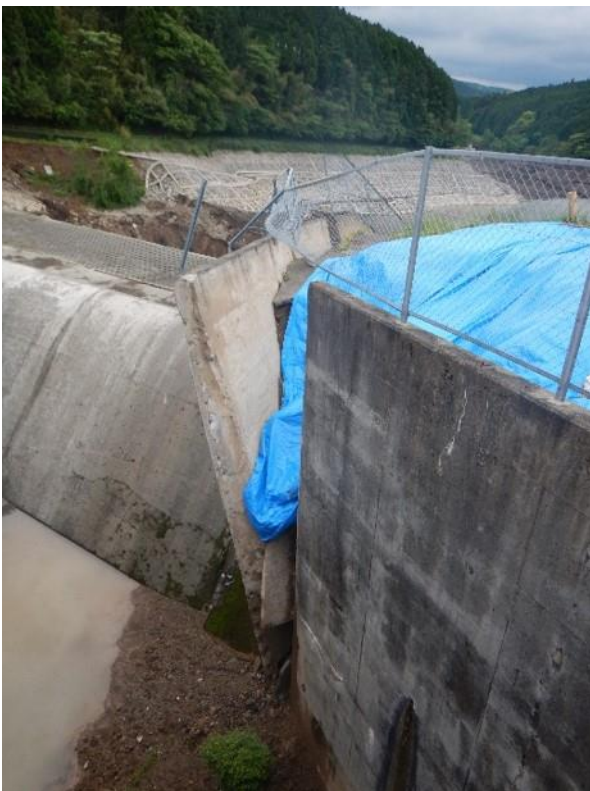
Photo 51: Close up of the damaged spillway of the Ookirihata earth dam (N 32.8414; E 130.9317).
