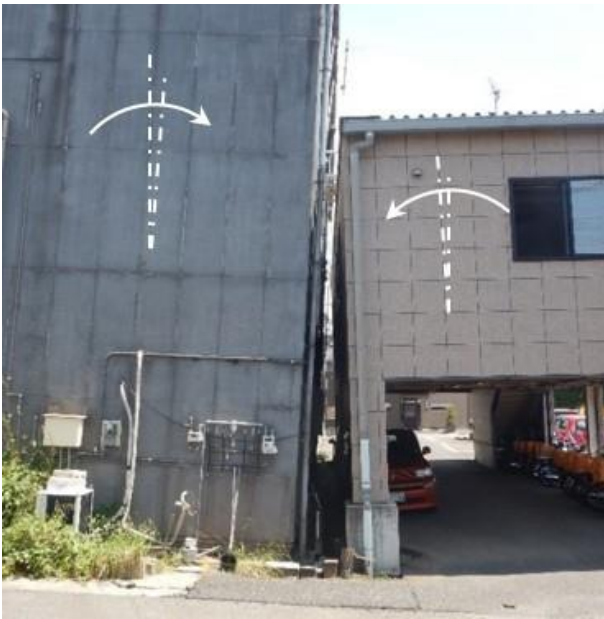
Photo 22: Liquefaction-induced tilting of two residential buildings in Kumamoto City (N 32.7600; E 130.6829).
