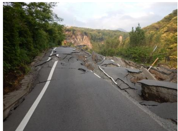
Photo 45: Severe disruption to approach embankment due to the collapse of underlain columnar jointed bedrock (N 32.8744; E 130.9827). See also Photo 18.
