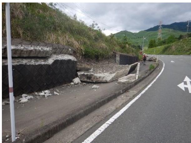
Photo 26: Fault rupture-induced collapse of a concrete facing unreinforced wall near the Ookirihata earth dam in Nishihara Village (N 32.8413; E 130.9317).
