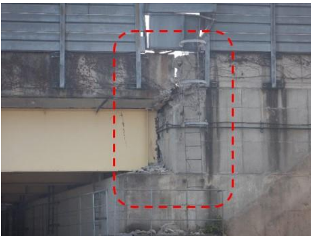
Photo 41: Punching of I-shape girder ends into the abutment wall caused shearing of back wall (N 32.7789; E 130.7943).
