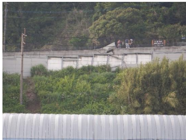
Photo 33: Good performance of a retaining wall with EPS block backfill (N 32.8792; E 130.9833).
