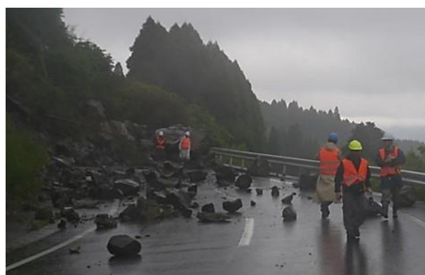
Photo 19: Typical rock fall on the road near the Tochinokibaru hot spring (N 32.8746; E 131.9884).
