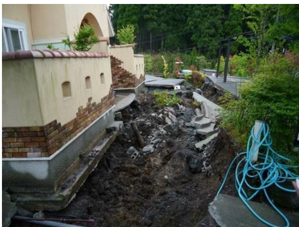
Photo 11: Translational slide / slump at Tokyu Country Town, Aso. About 40 houses were affected by landslide movement (N 32.8796; E 131.0030).
