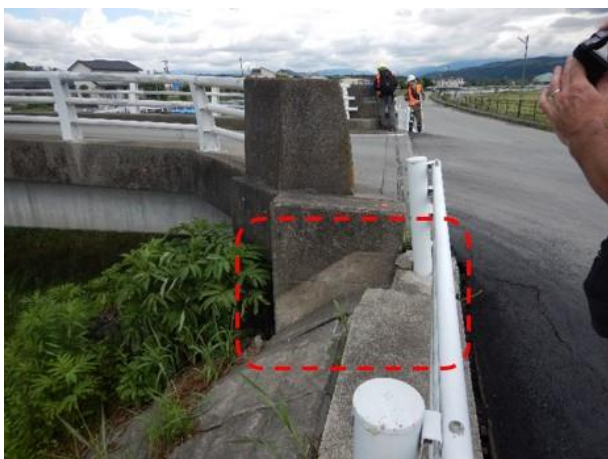
Photo 35: Typical settlement of short span concrete bridge approaches observed in Mashiki Town (N 32.7830; E 130.8085).
