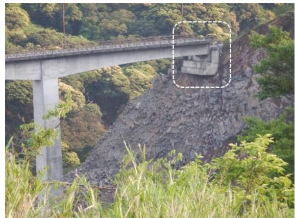
Photo 44: Abutment foundation failure due to the collapse of underlain columnar jointed bedrock (N 32.8770; E 130.9840). See also Photo 18.
