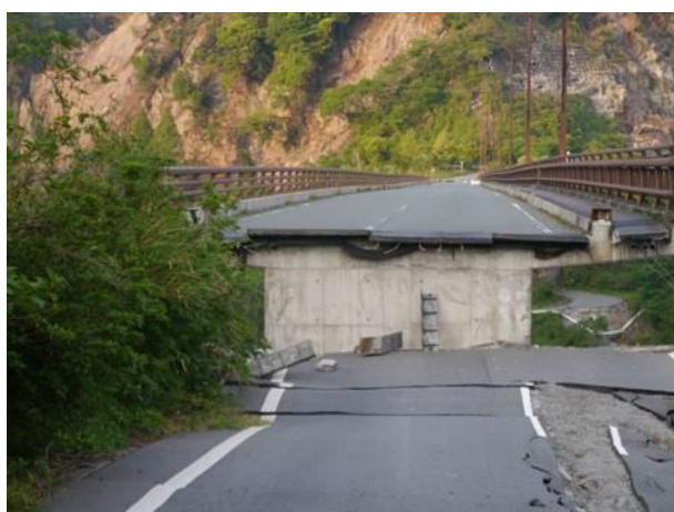
Photo 18: Displacement of the road bridge abutment. The displacement resulted from loosening and toppling of the jointed rock mass supporting the abutment foundation (N 32.8764; E 131.9827).
