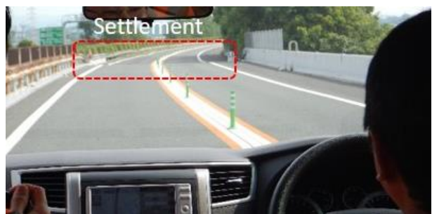
Photo 49: Settlement of expressway on embankment (N 32.7789, 130.7939).
