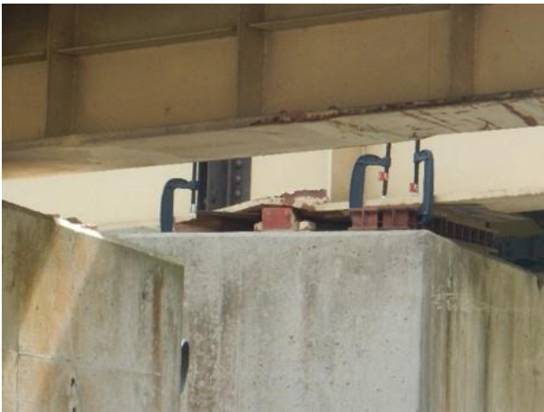
Photo 40: Local buckling of girder bottom. The girders were re-levelled temporarily with steel plates either side of original bearings (N 32.7790; E 130.7939).
