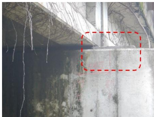
Photo 38: A two span bridge jumped 300 mm laterally off its bearings (view of the bearing) (N 32.7864; E 130.8186).
