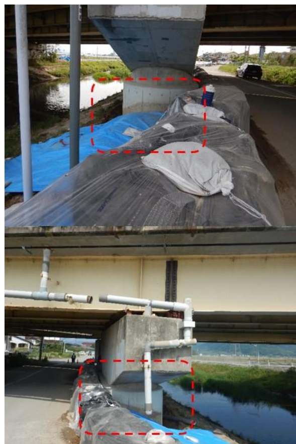
Photo 39: Ground settlement around piers of a long span steel girder bridge observed in Mashiki town (N 32.7787; E 130.79.39).
