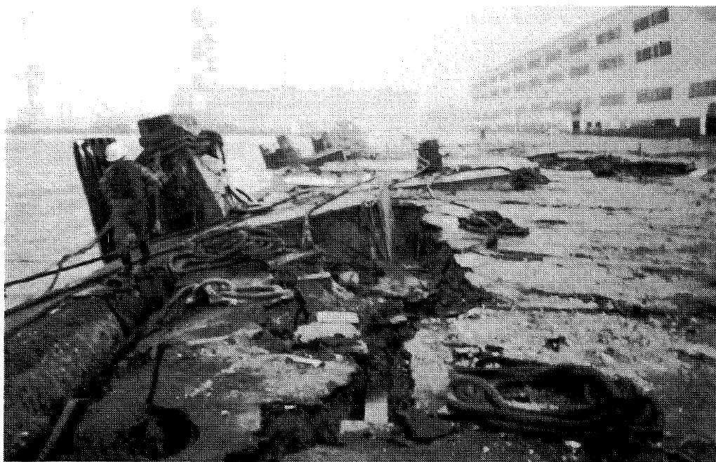
Figure 5 Hakodate Port - Liquefaction damage
