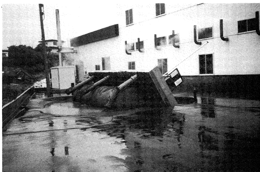
Figure 4 Liquefaction and uplifting of 20 m 3 storage tank (one third full)
