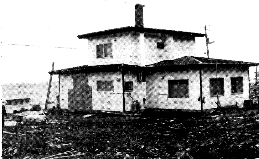
Figure 9 Timber framed house near Inaho which survived the tsunami which appeared to be about 3-4 m high. Note the puncture damage to the external sheathing due to debris.
