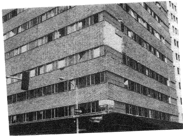
FIGURE 4 BRICK VENEER FAILURE
