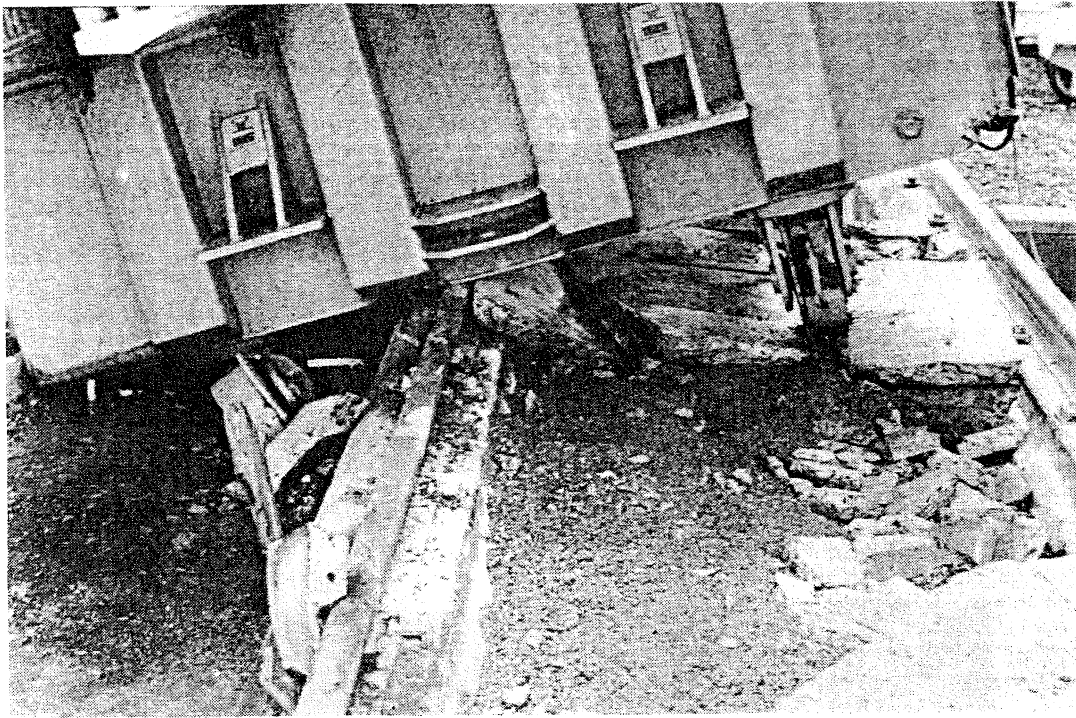
FIGURE 7 220KV TRANSFORMER AT EDGE CUMBE OFF THE RAILS
