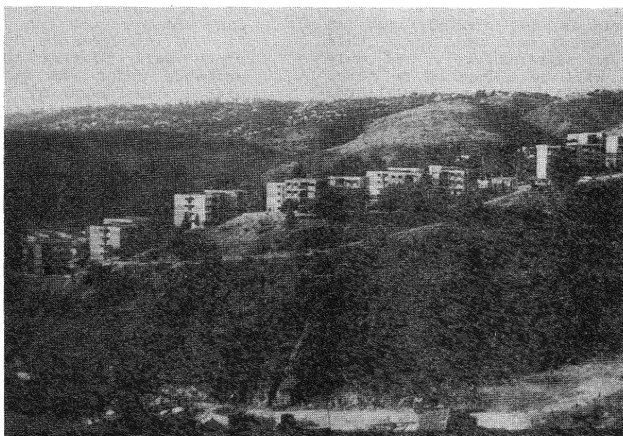
Figure 3. Topographical focusing appeared to have worsened the shaking for the buildings on this ridge, Villa Canal Beagle, Vina del Mar.
