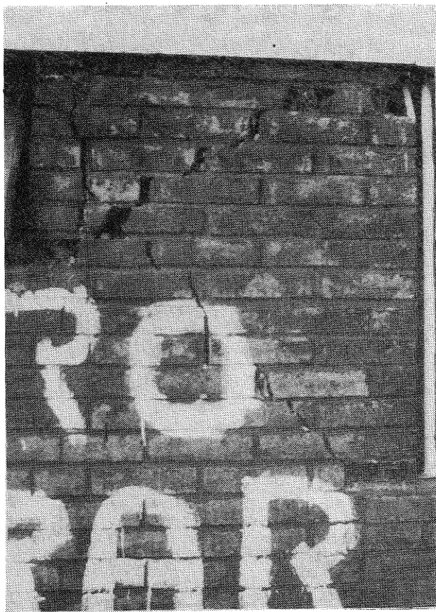
Figure 1. Shear cracks in reinforced brick walls, Villa Santa Carolina, Santiago.
