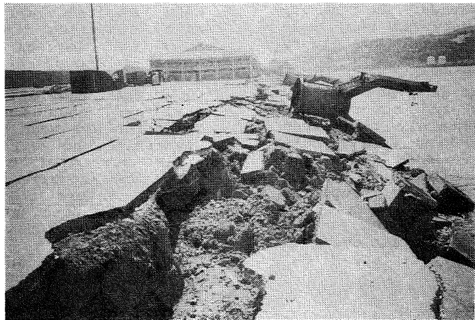
Photo 22. Subsidence of reclamation and complete collapse of retaining wall wharf leading to crane toppling.
