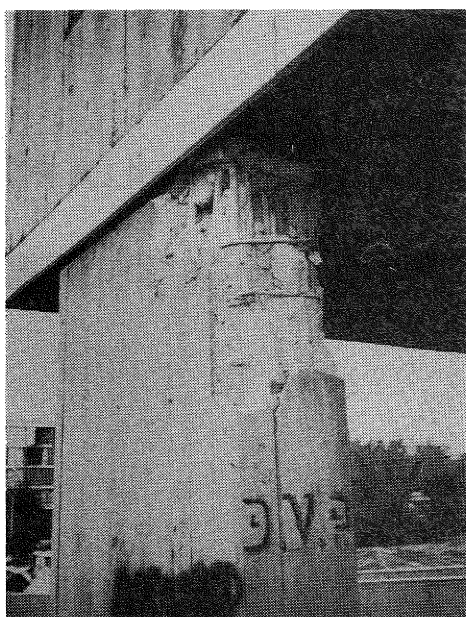
Photo 11. Left-hand (east) column/wall joint.
