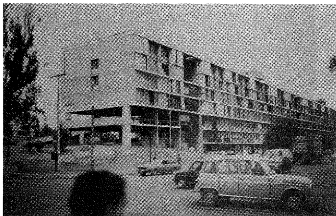
Photo 10. North end wall showing shear wall transition to columns.
