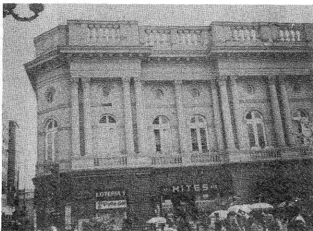
Photo 19. Badly damaged parapet, cracking near corner of building and around window arches.
